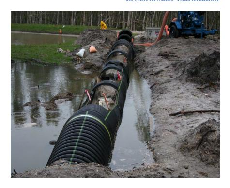
The project had been trying to control the discharge of turbid water by treating the lakes on a monthly basis, with poor results. It was decided to install a continuous flow-through treatment system to treat the turbid water before discharge off site. A split pipe treatment system was designed to clarify the water before discharging into state waters.
