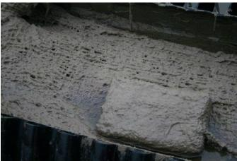
The split pipes were lined with jute matting, which provided surface area for the flocculated particulate to adhere to. The clarified water was then discharged off site.
