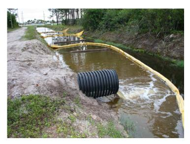
Above, Right: The sediment was reacted with the Floc Logs, binding the particles together and attaching them to the jute matting in the split pipe system.
